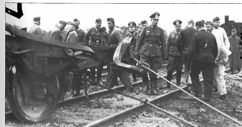
German pioneers working to convert the wide Russian-gauge railway to the narrower European standard. As the Wehrmacht advanced, this sort of work would be vital as the road system in southern Russia was primitive at best and so the railway would be vital in keeping the forces supplied. (Nik Cornish Library)
